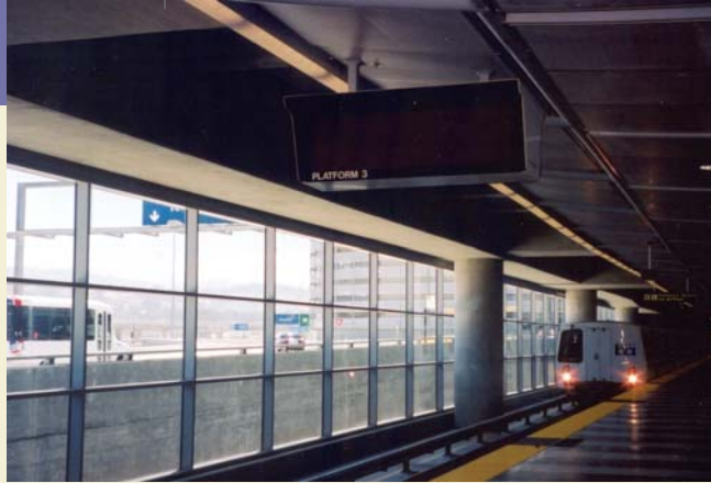
Line Extensions Project, San Francisco, CA (BART)
